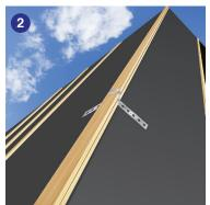
Build up the ridge batten using 25mm thick battens to the required height, usually two battens are sufficient for most profile tiles. Secure the battens in place using the stainless steel batten straps provided. Where Verge Units are to be installed, the ridge batten must extend beyond the ridge by 30mm at each gable end.
